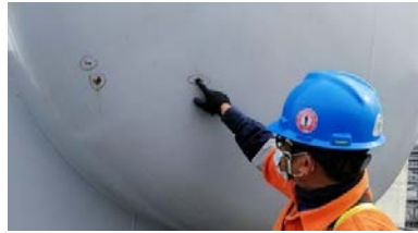
Figure 6. Coating inspection on asset condition. Source: Author collection
